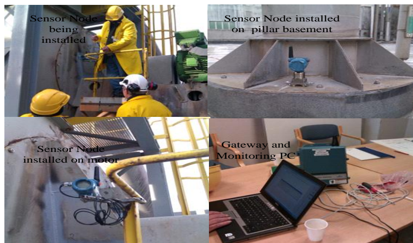
Figure 5.4: Engineers busy on random installation of wireless HART in Yara, Porsgrunn
